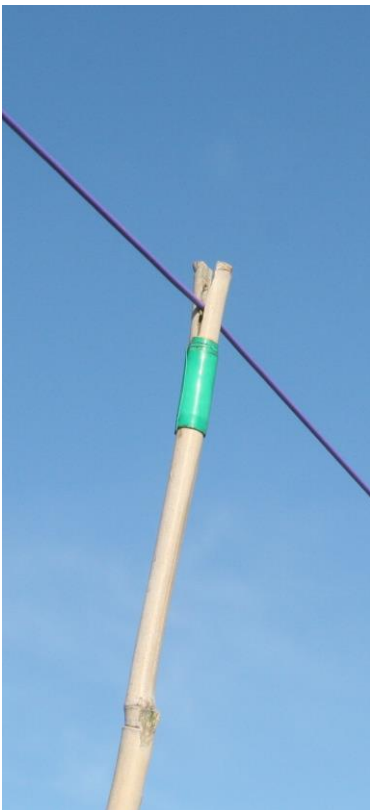
Fig 7a: Bamboo every 5-10m Fig 7b: Intermediate 40mm x 40mm Fig 7c: Ends 75mm x 75mm
